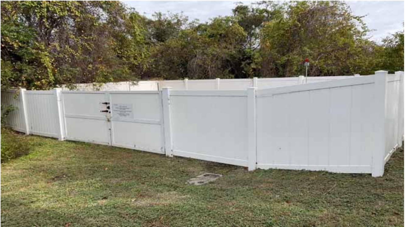
Fence - Lift Station
