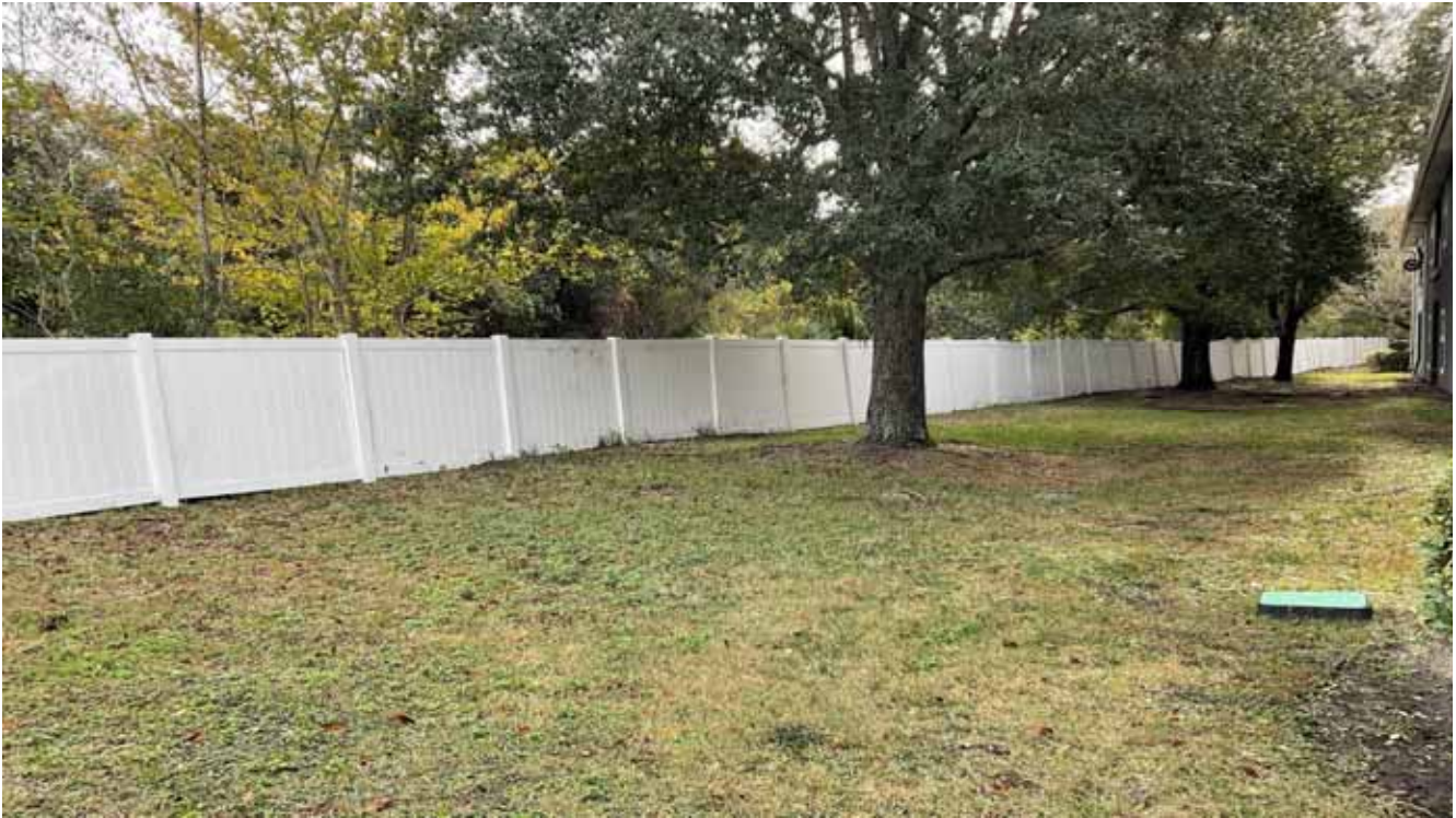
Fence - Property Line
