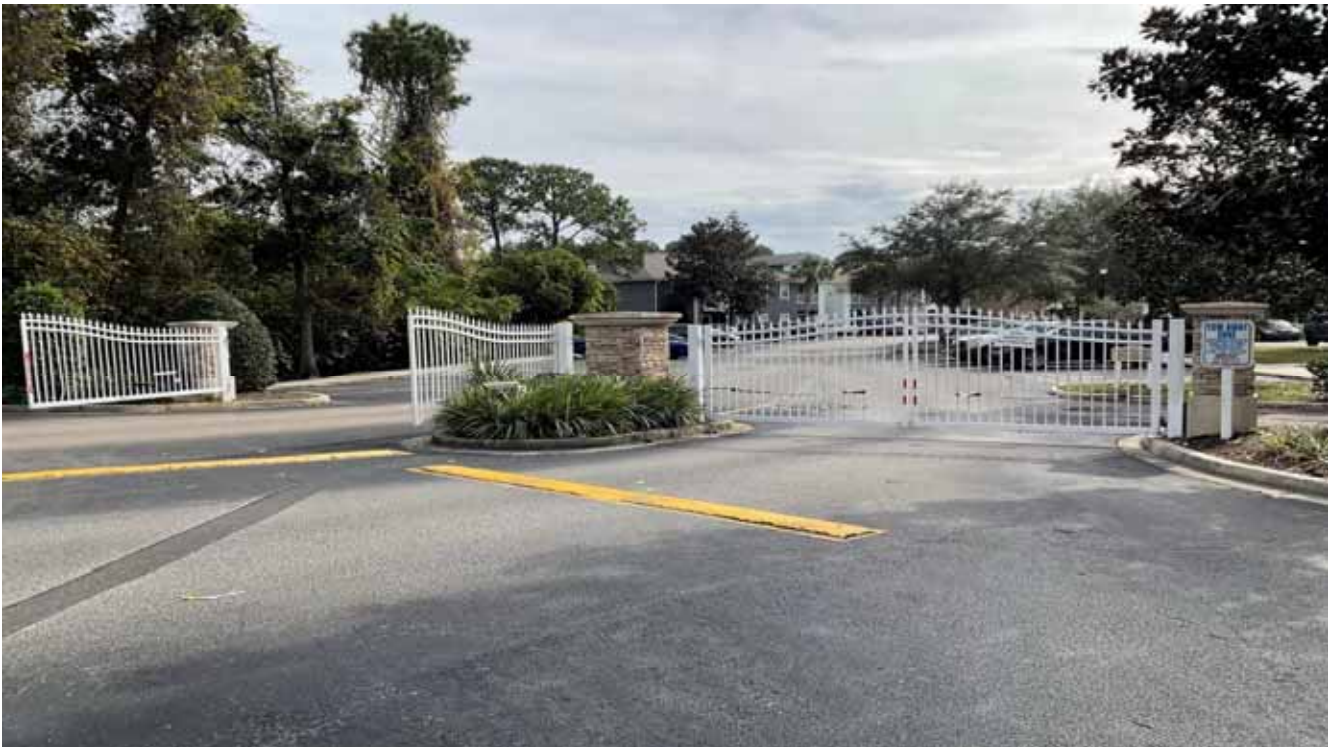
Entry Gate System
